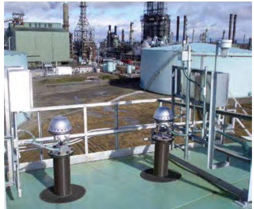
Figure 9.3: Tank redundancy is accomplished with dual tank gauges and separated communication layers - wired and wireless.
