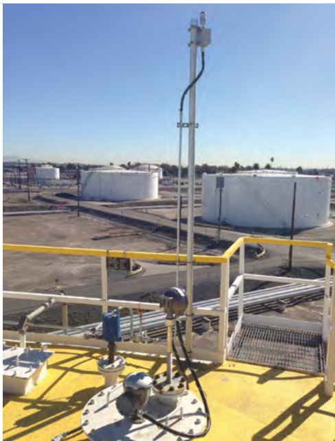
Figure 9.8: Antenna connected to tank devices.
