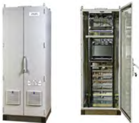
Figure 9.5: A tank gauging system cabinet.
