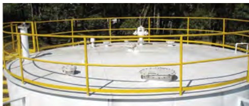
Figure 2.14: Fixed roof tank openings.
