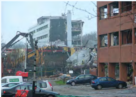
Figure 10.1: Property damage after the accident at Buncefield.
